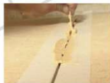
Pre grout the joint
