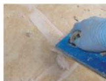
Forcing grout deep into grout joint
