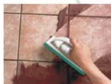
Clean off with water and by scrubber
